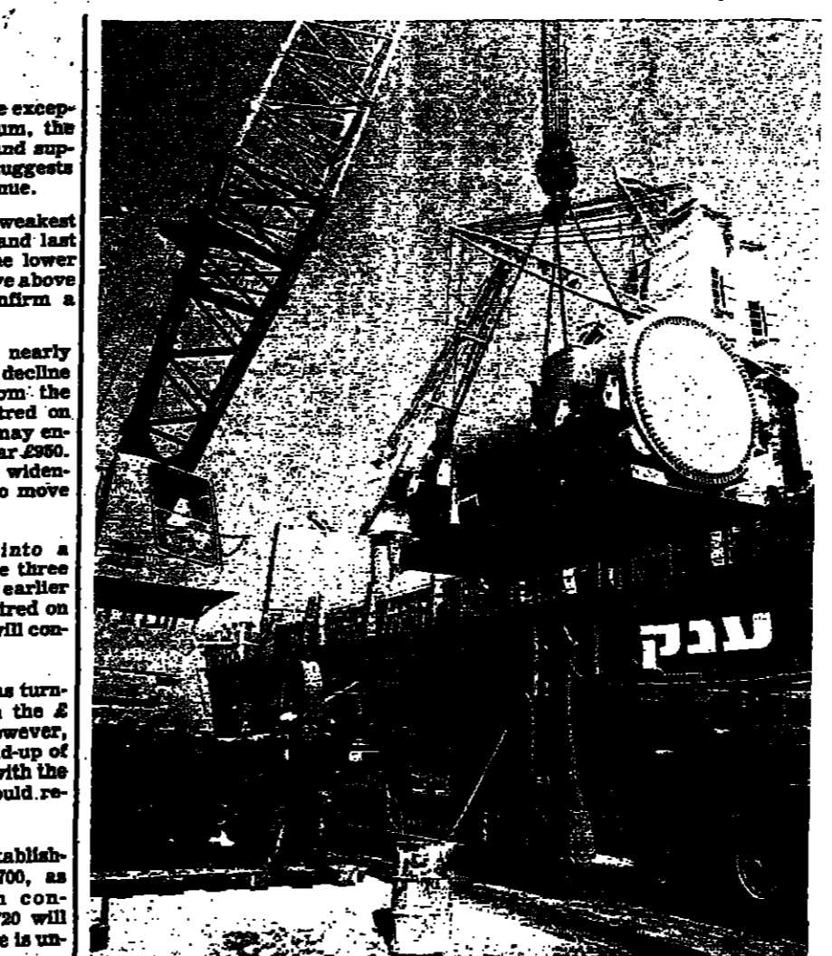
This 250-ton generating unit destined for the new Hadera power station was off-loaded from a freighter at Haifa port yesterday. The giant dock-side crane is seen lowering it gently onto the special multi-axle Zam land transporter.
